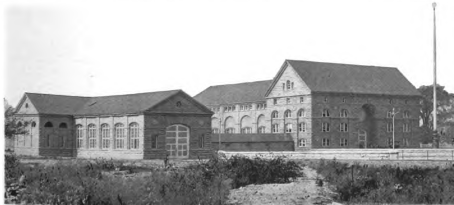
HYDRAULIC POWER STATION—NIAGARA FALLS POWER CO.
