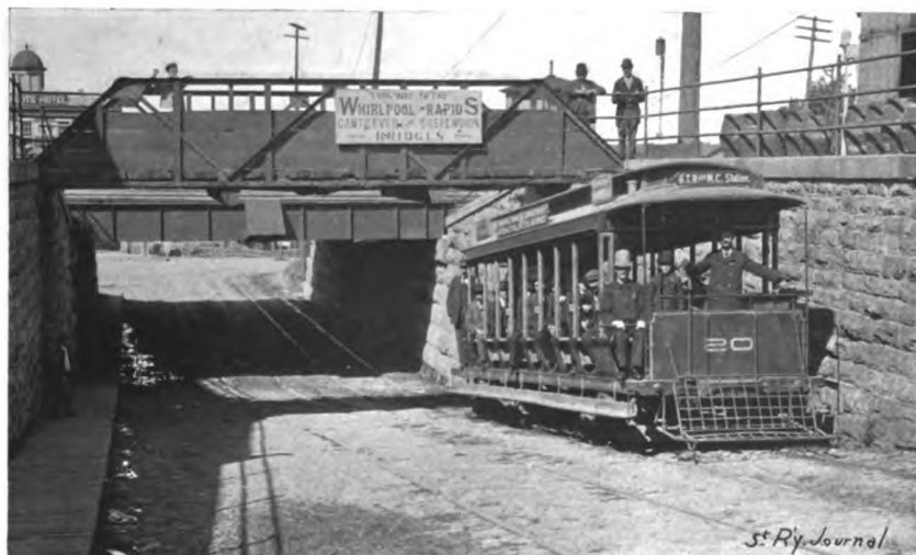
13 PER CENT GRADE IN CUT—NIAGARA FALLS & SUSPENSION BRIDGE RAILWAY.
