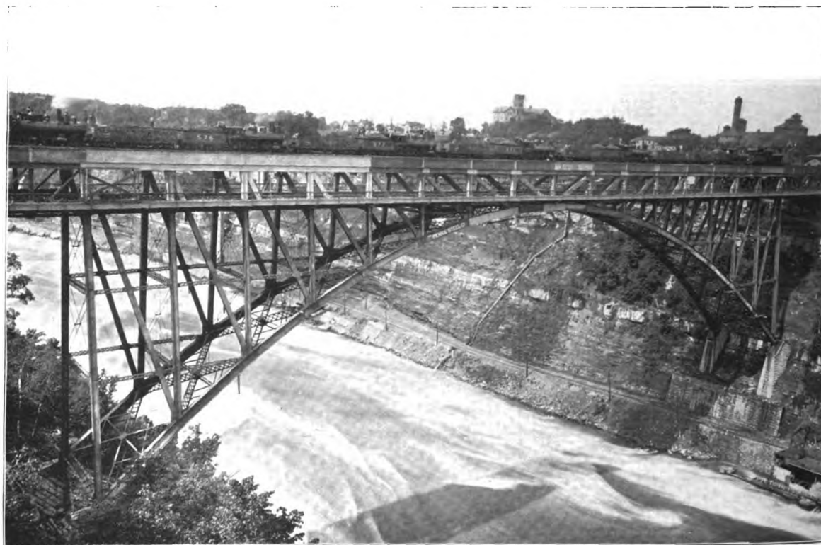
SPAN GIRDER BRIDGE ACROSS NIAGARA RIVER.
